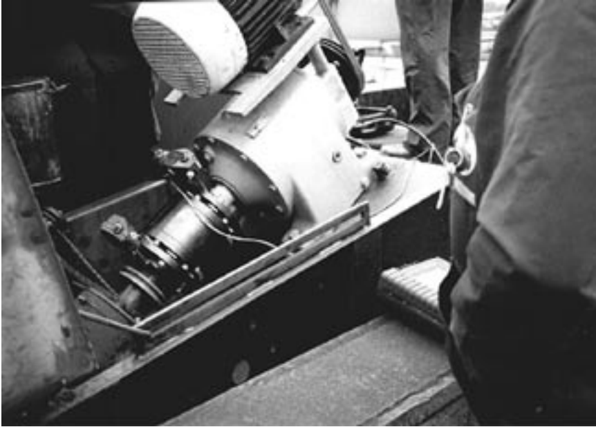
Water Treatment Installation
